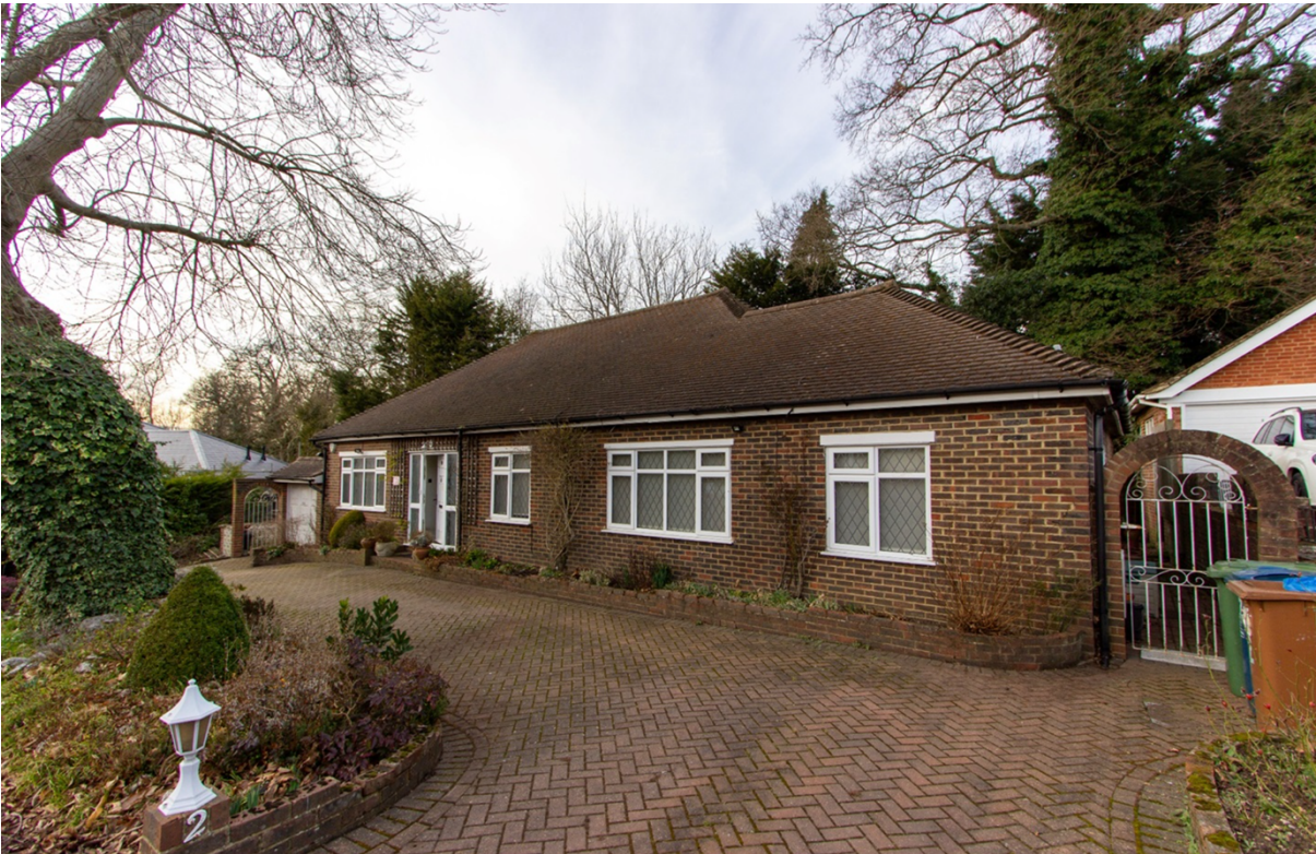
Front elevation and eastern side boundary with no. 1
